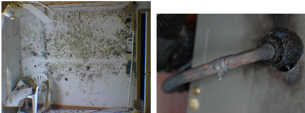
Figure 4.3 Photos of defective Chinese drywall and corrosion it's caused to pipework
