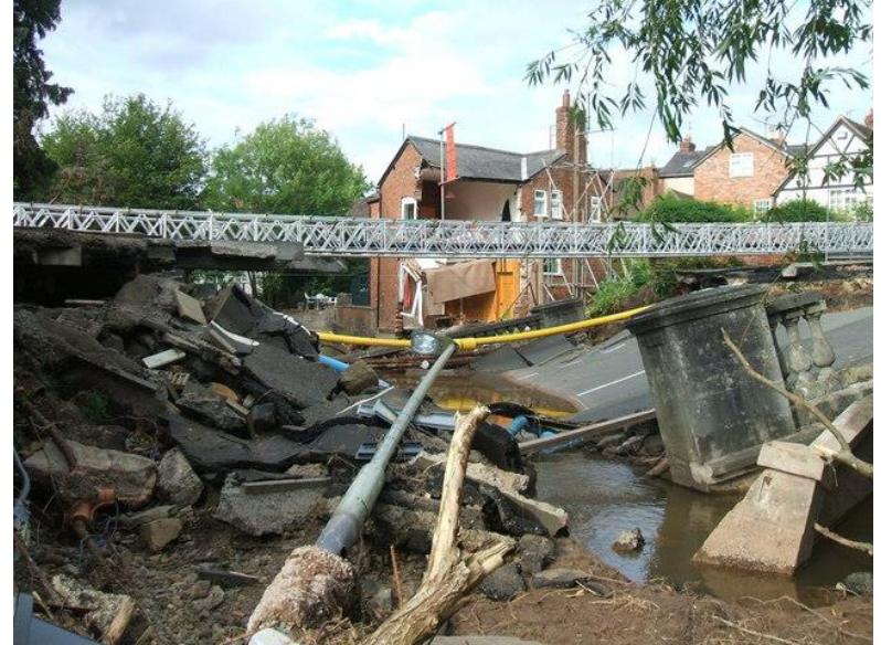
DI Wyman / Flood Damage / CC BY-SA 2.0
